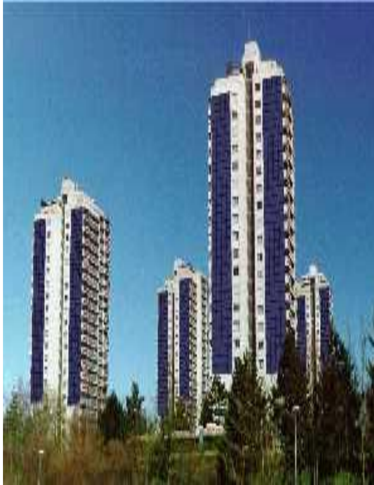
SunSlate Building-Integrated Photovoltaics (BIPV) commercial building in Switzerland
