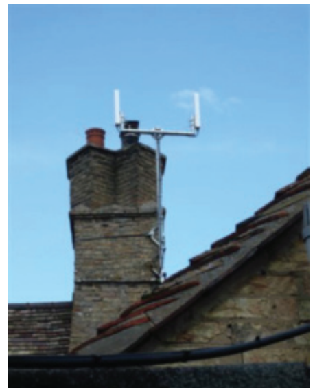
Figures 03 & 04: TVWS antennas, installed at the ADC theatre and at one of the pubs Photo: CSR
