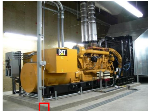
2.5MW Generator ~180 Gallons/hour
